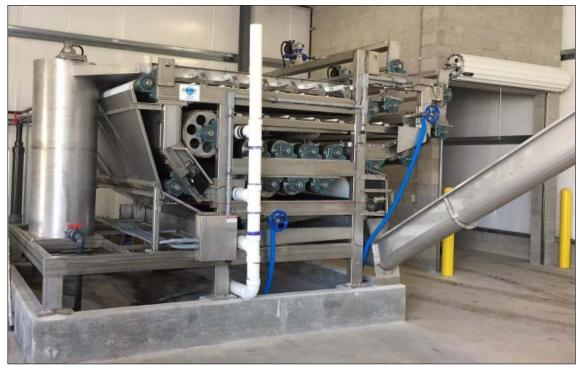
The OR-TEC Gemini Series Belt Press is a double belt system ideal for the medium to large size W.W.T.P. This press combines a gravity drainage zone, a low pressure zone and high pressure shear zone to provide a large dry solids throughput and an excellent final cake. The system can be customized to the clients needs with a full range of ancillary equipment from sludge pumping to dry cake conveying
